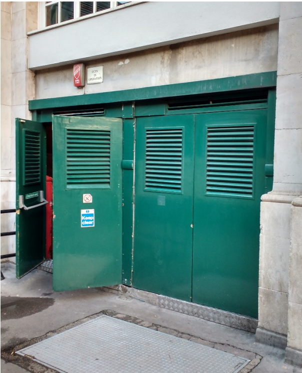
Secondary Entrance on Tavistock Court (right)
